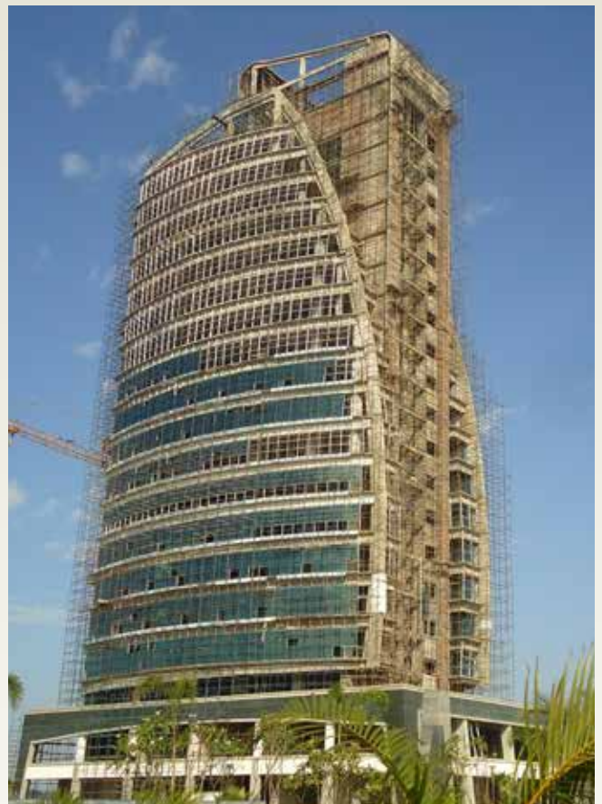
India Trade Tower, New Chandigarh
