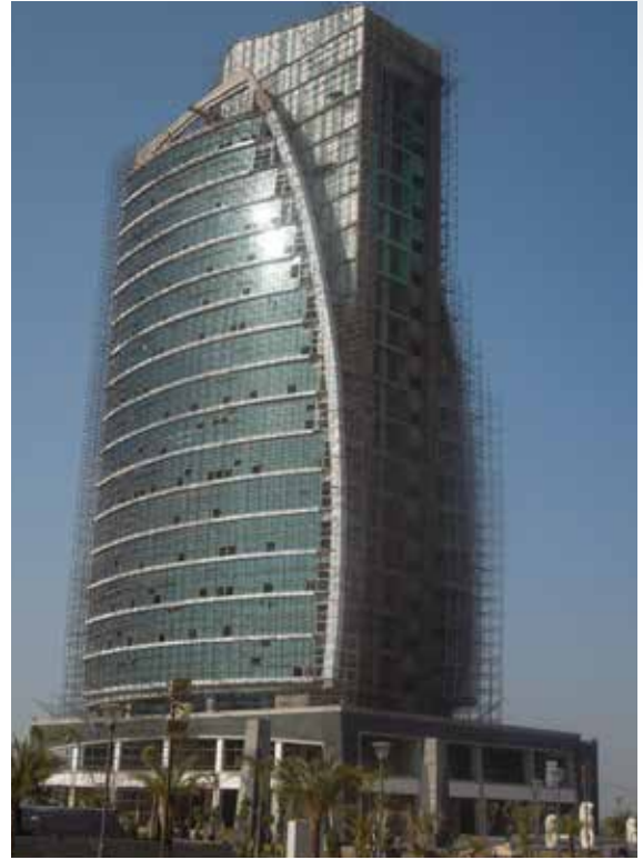
India Trade Tower, New Chandigarh
