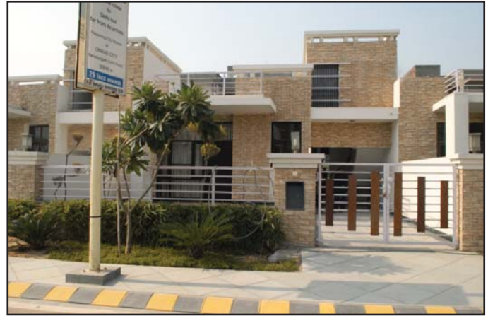
Villas at Omaxe City, Bahadurgarh (Expandable Villas )
